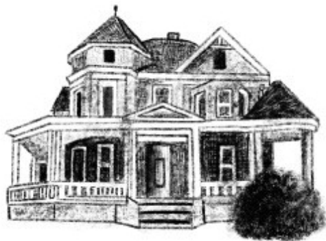
Boulder County Poor Farm, late 1800s & early 1900s
